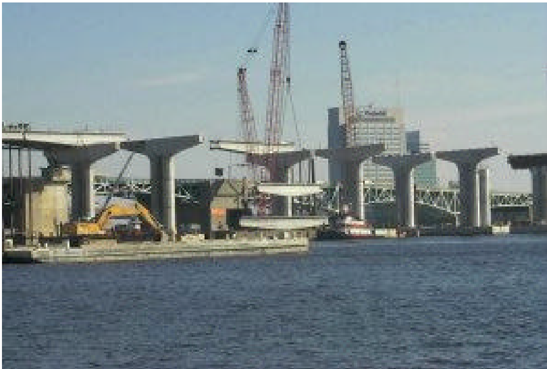
Replacement of the Fuller Warren Bridge in Jacksonville.
