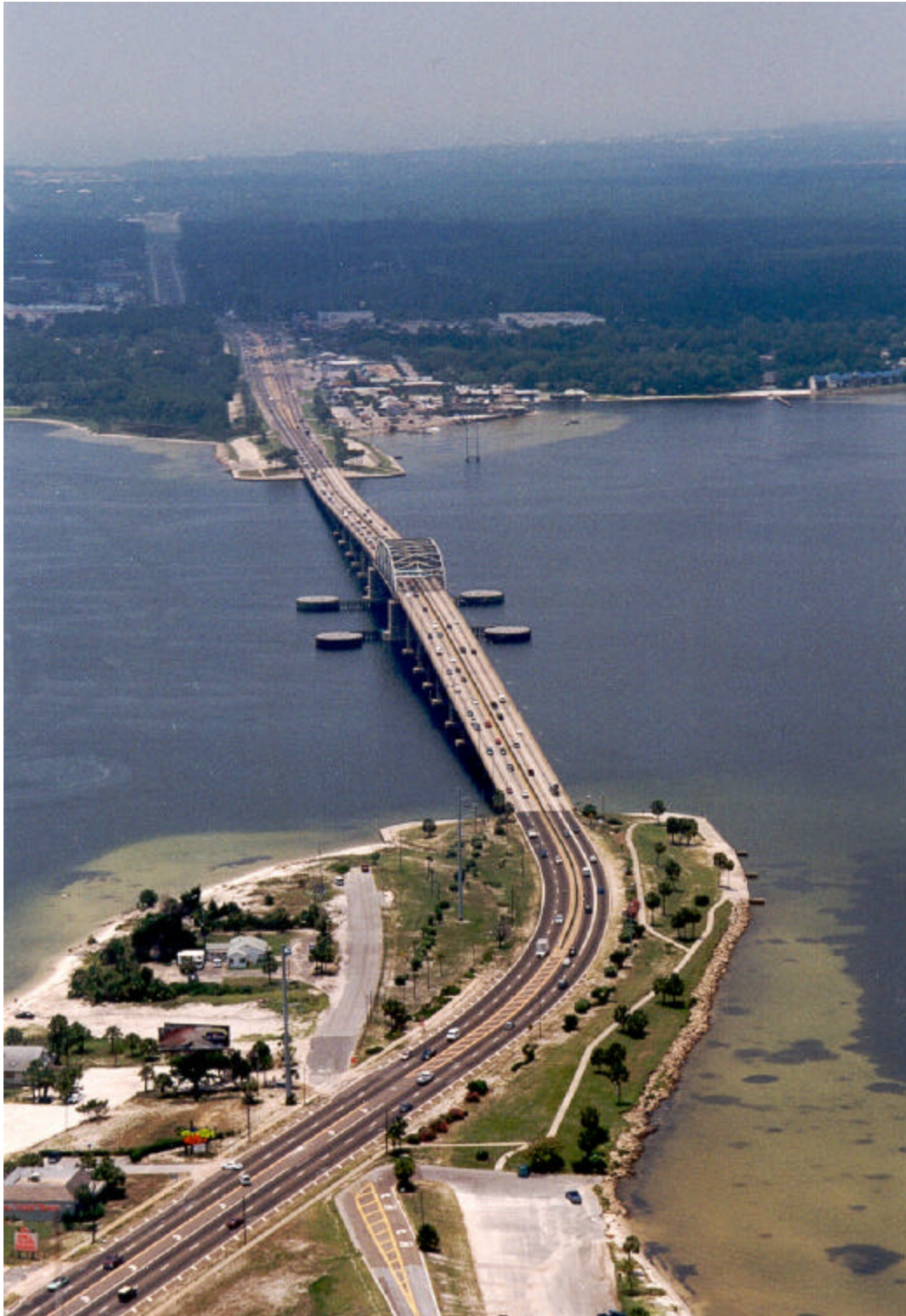
Hathaway Bridge, Panama City.
