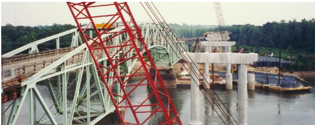
Apalachicola River Bridge Construction – Highway 20.
