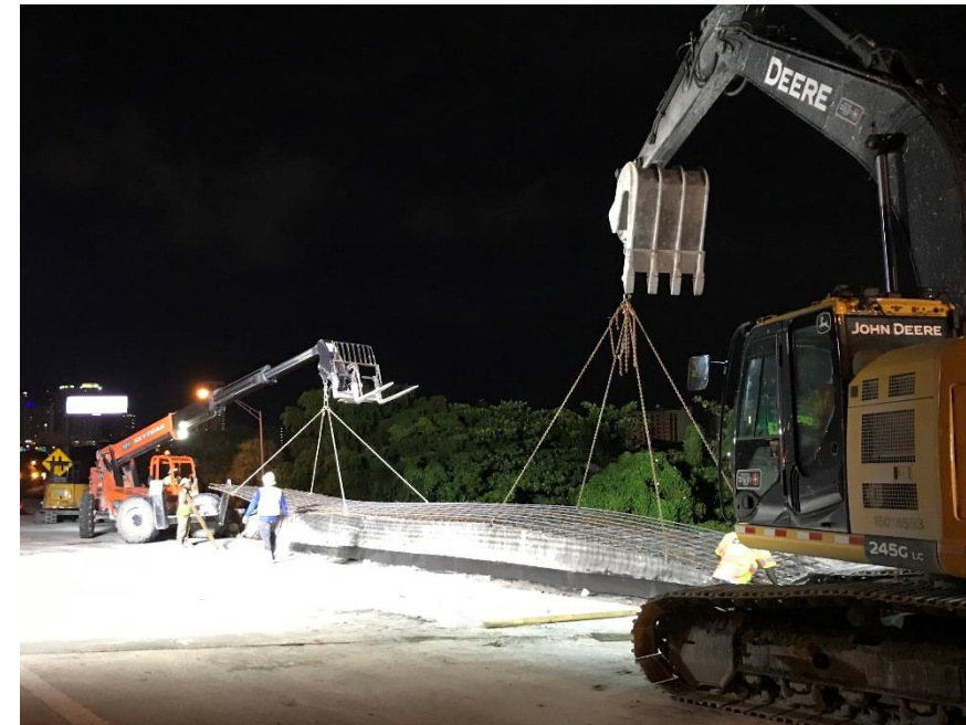
Bridge approach slab replacement
