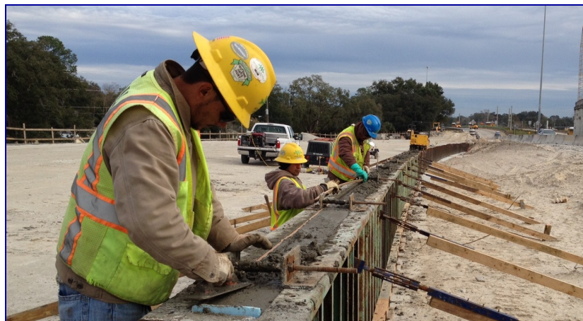
Rigid Barrier Wall Concrete Finishing
