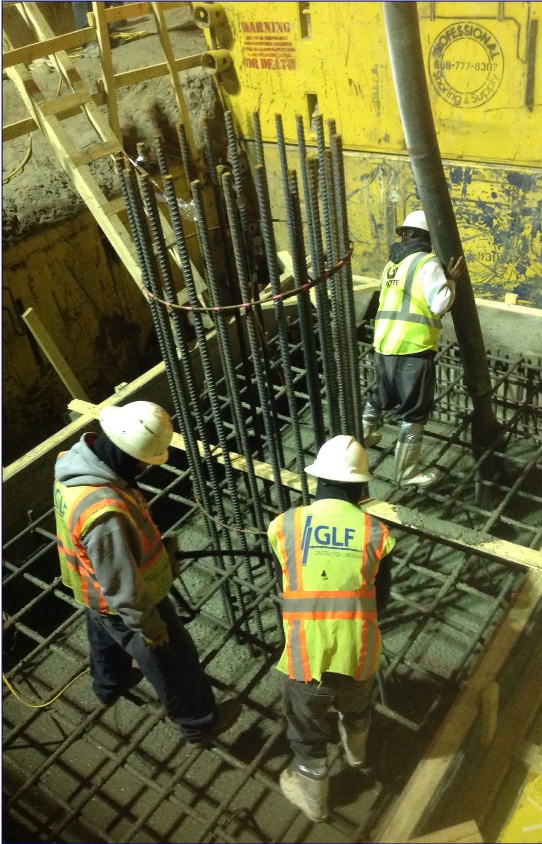
Wilsky Bridge Footer Mass Concrete Pour – Turnpike
