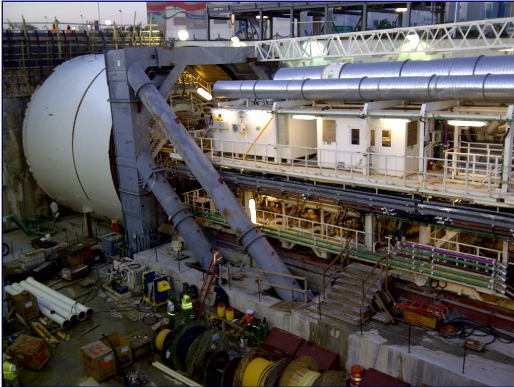
View of Tunnel Boring Machine Trailing Gear
