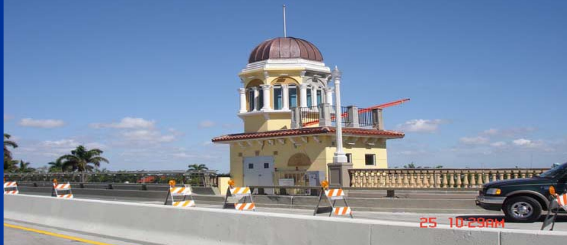
New Gatehouse with Copper Domed Roof on Hollywood Boulevard Bascule Bridge-District 4
