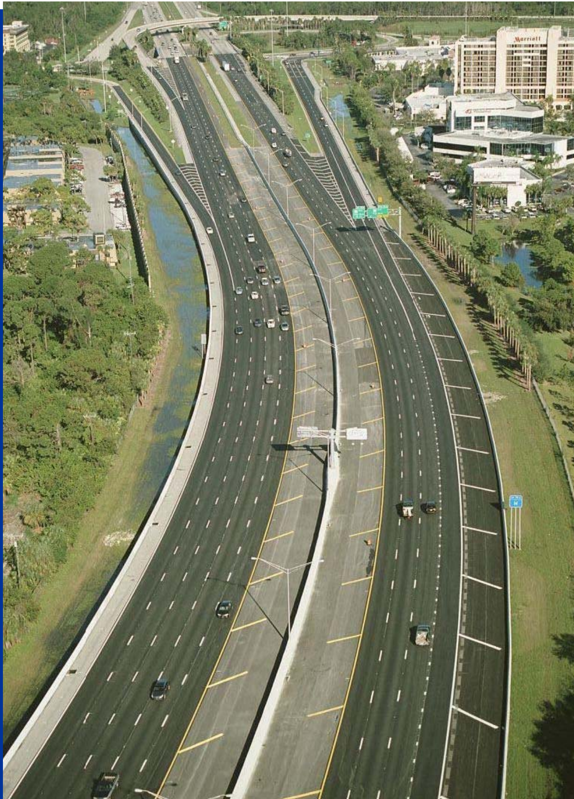
A district 4 Design/Build project to add lanes (from 6 to 8 lanes) and reconstruct I-95 from north of Blue Heron Boulevard to PGA Boulevard (2.581 miles).
