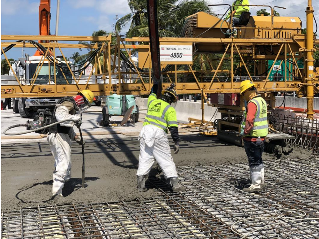
State Road 5 – Cow Key Channel Bridge Deck Pour District 6
