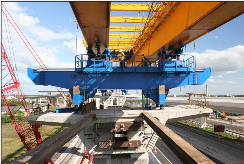
Bridge Gantry being used on the Cross-town Connector project.
