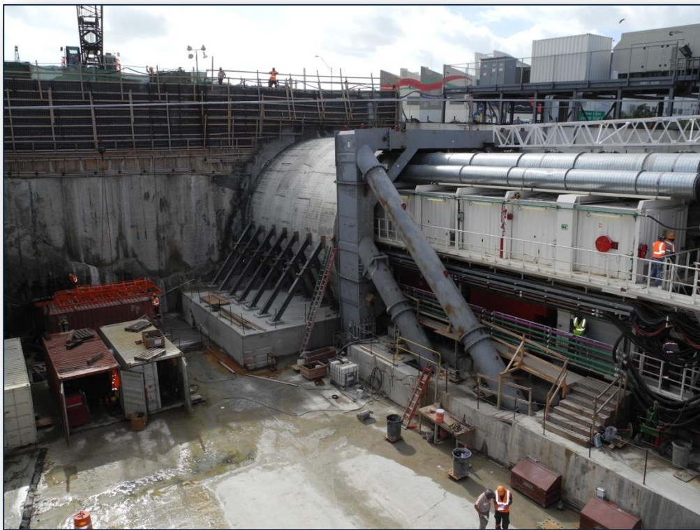
Port of Miami tunnel boring machine.
