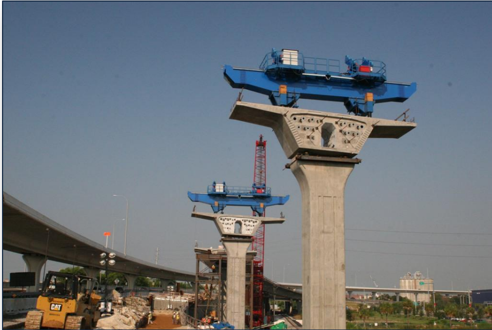
Piers 7 and 6 for the Cross-town Connector project in Tampa.
