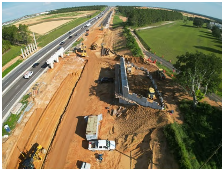
Florida's Turnpike Mainline/State Road 91 Widening (Florida's Turnpike Enterprise)
