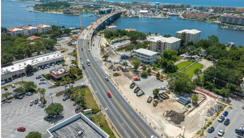
Brooks Bridge Replacement Project (District 3)
