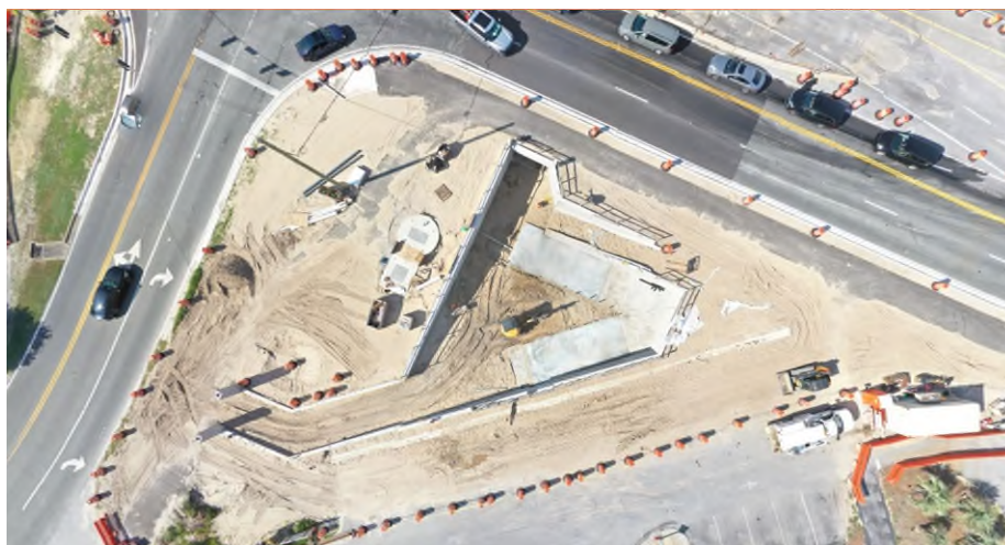
U.S. 98 Pedestrian Underpass at Inlet Beach (District 3)
