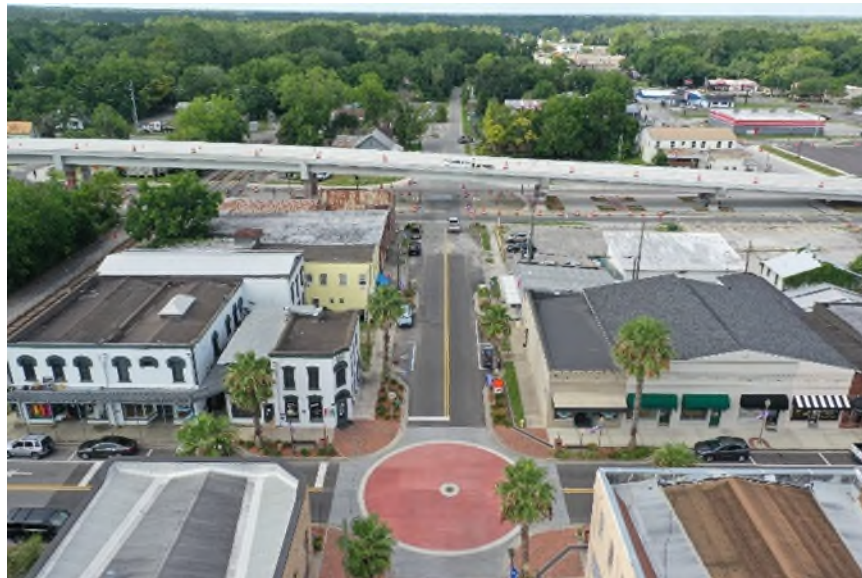
Starke Railroad Overpass (District 2)
