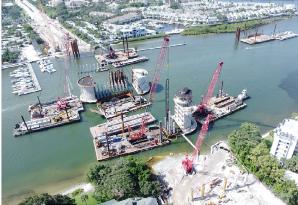
Jupiter US 1 Bridge Replacement (District 4)
